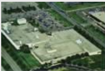
Global headquarters of McQuay (Minneapolis, USA)
