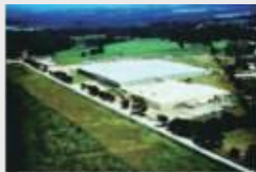
McQuay Auburn Factory, USA
